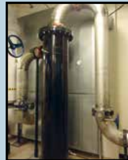
Protecting heat exchangers, Nevada USA
