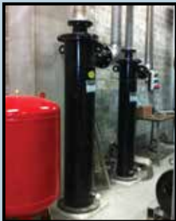
Cleaning chilled water, Axima Belgium
