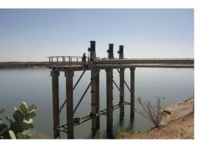
Vertical line-shaft pumps enable considerable savings to be achieved in the construction of pumping stations.
