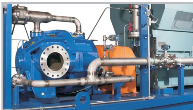
NASH HP-9 Flare Gas Recovery Unit
