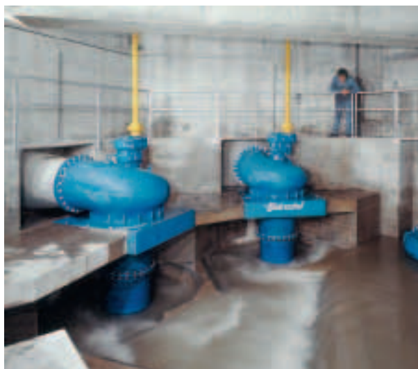
Sewage lift station with vertical installation and the PREROSTAL® flow regulating system.
