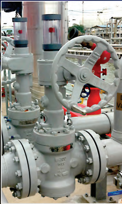
OmniSeal® plug valves in service
