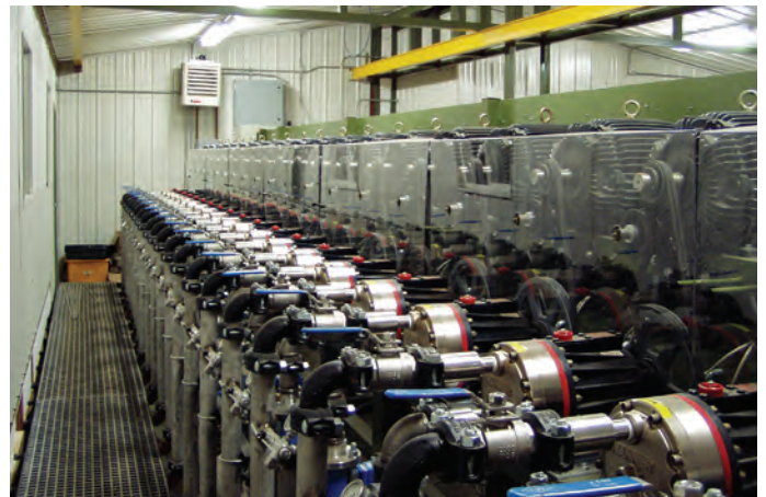
Hydra-Cell pumping shear-sensitive polymers for enhanced oil recovery.
