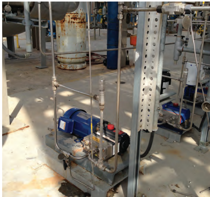
Hydra-Cell pumping ethanol-based fluid for making jet fuel.
