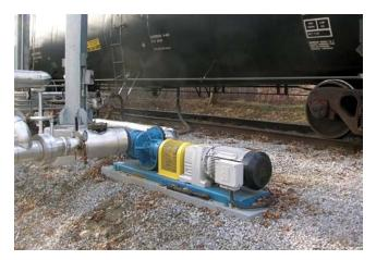
Viking internal gear pump in a railcar unloading application.
