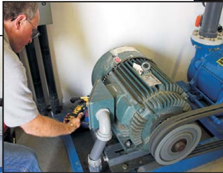
Left to right: Checking connections, checking amperage and performing a borescope inspection
